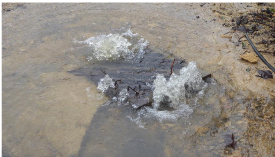
Photo 8: Drainage Overflow, Crudwell
