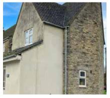
Figure 20: Stone with render on one wall.
