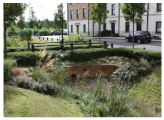
**Figure 49:** Example of swales and a dam integrated with a crossing point, elsewhere in UK.
