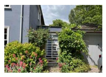
Figure 47: Heat pump screening at the front of a dwelling.
